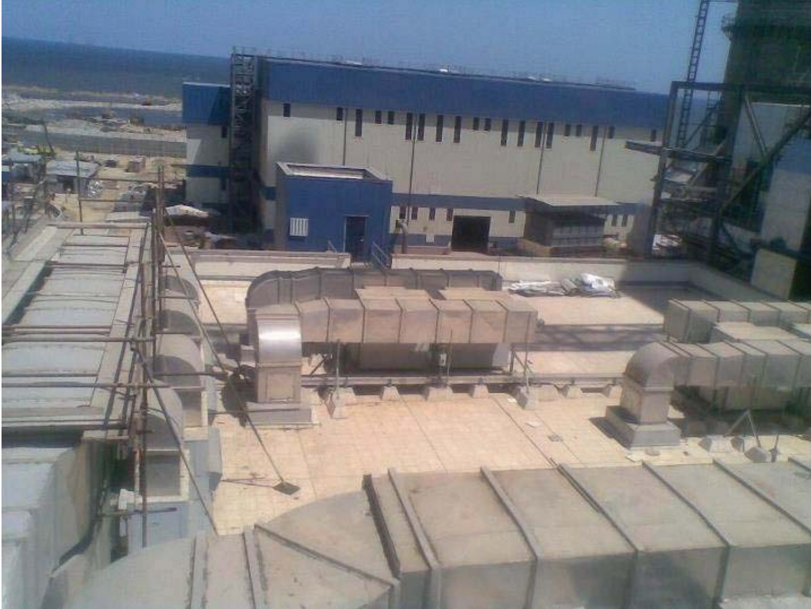
Abu Qir Thermal Power Plant
