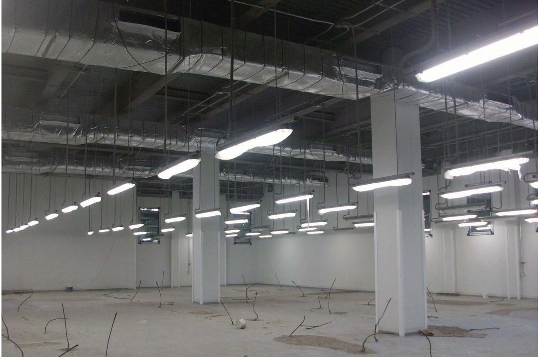
Abu Qir Thermal Power Plant Control Building
